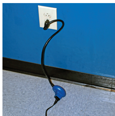
Load Tester plugged in-line with the device
