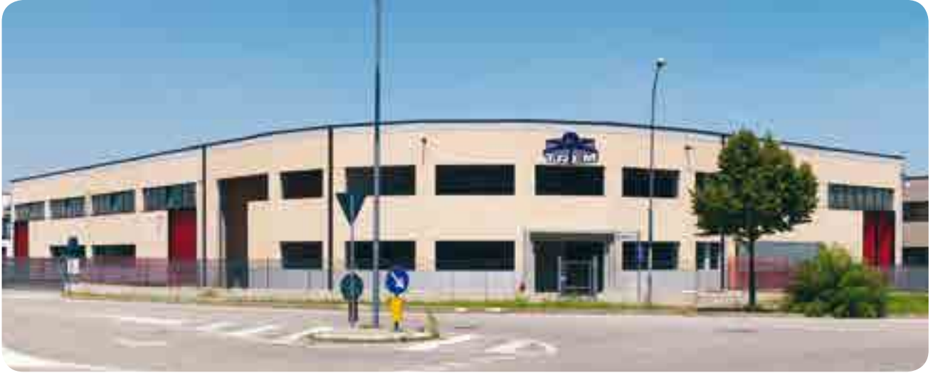
4 New plant (from south)
