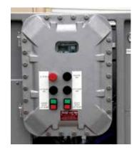
Explosion proof control box with E-stop and metallic cable glands; connected with armored cables
